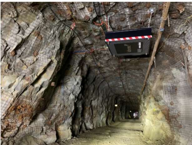
Figure 5 Ideon's Mine Muon Hub installed in a mine.
